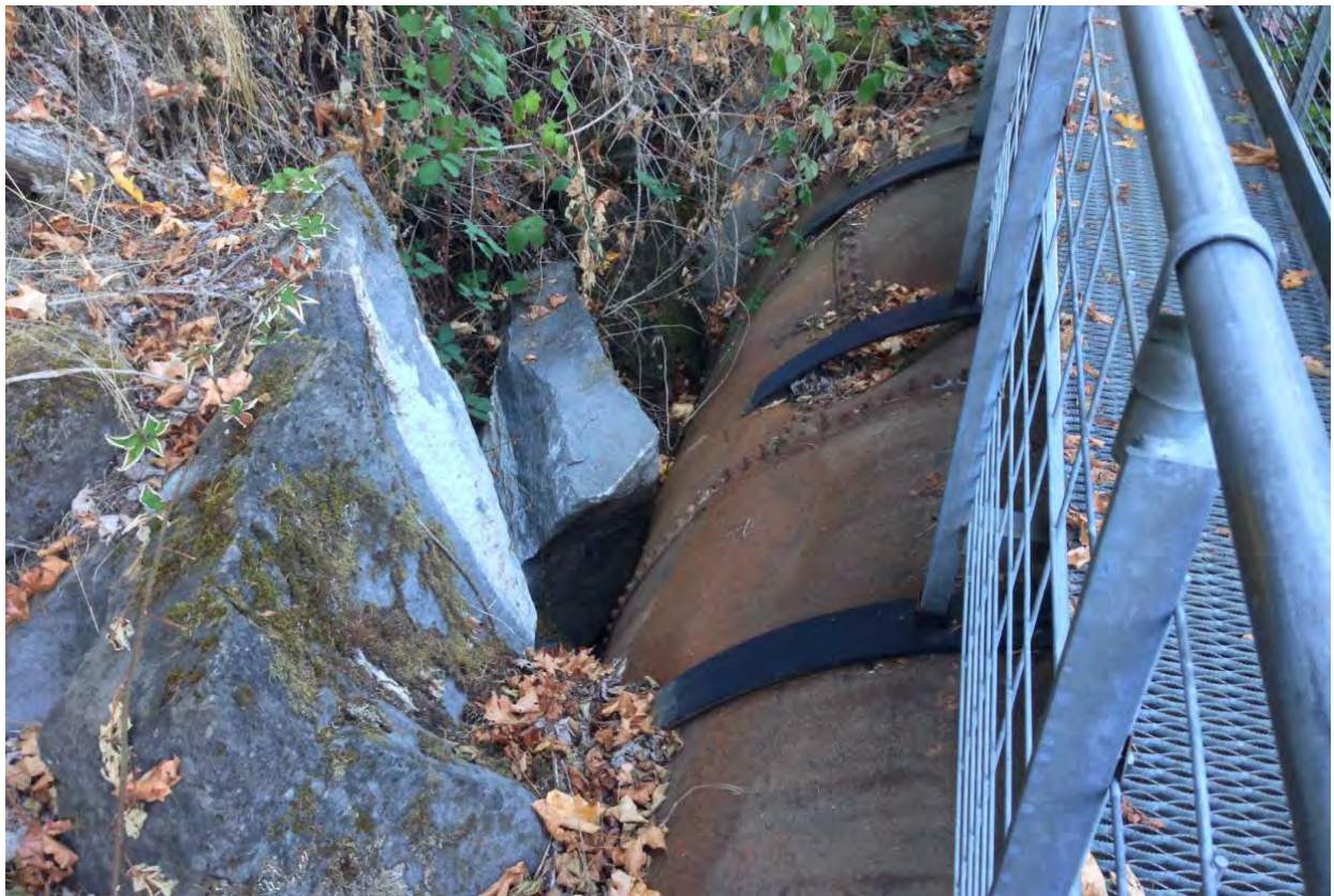
Figure 12: Dent from falling rock in welded steel pipe section.
