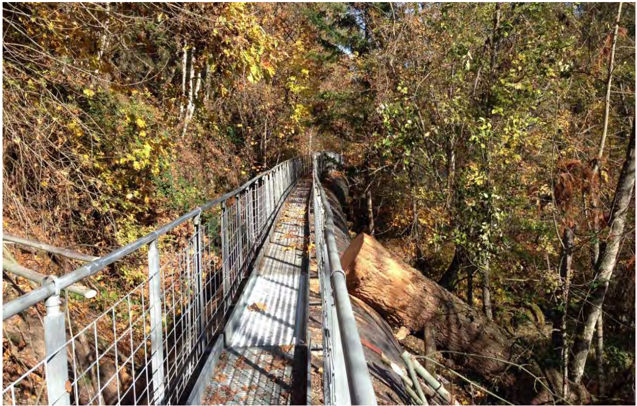
Figure 17: Looking downstream at the catwalk sections knocked off pipe. Top: Sept. 2015, from a point near the downstream end of the damages. Bottom: Nov. 2015, repair completed, from a point just upstream of the damaged sections.
