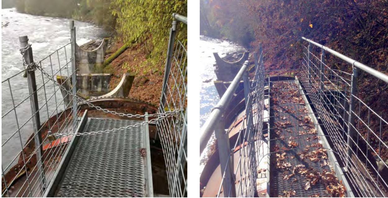
Figure 10: Left: Chain at the upstream end of the catwalk; view of pipe washout site. Right: Hog wire fence added to the end of the catwalk in November 2015.
