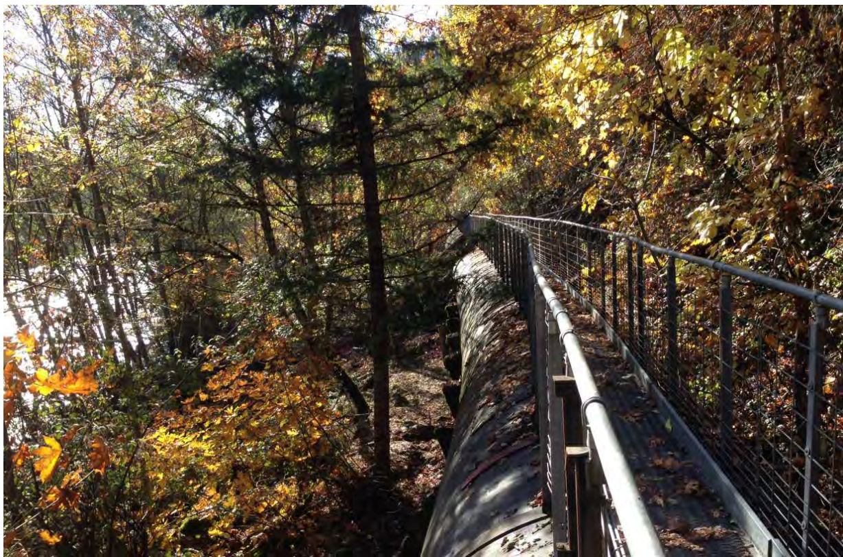
Figure 16: Looking upstream at the catwalk sections knocked off pipe. Top: Sept. 2015. Bottom: Nov. 2015, repair completed.
