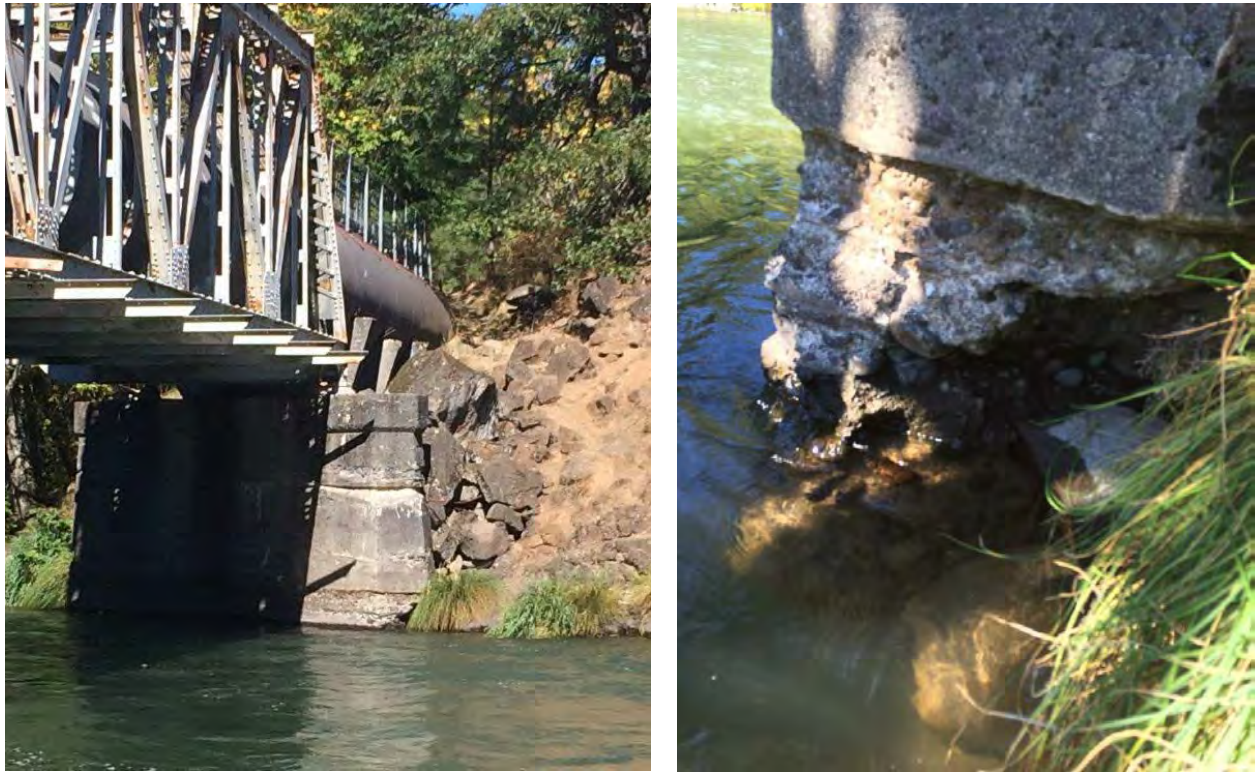
Figure 19: Photos from engineer showing erosion at base of pipeline bridge's northeast pier.
