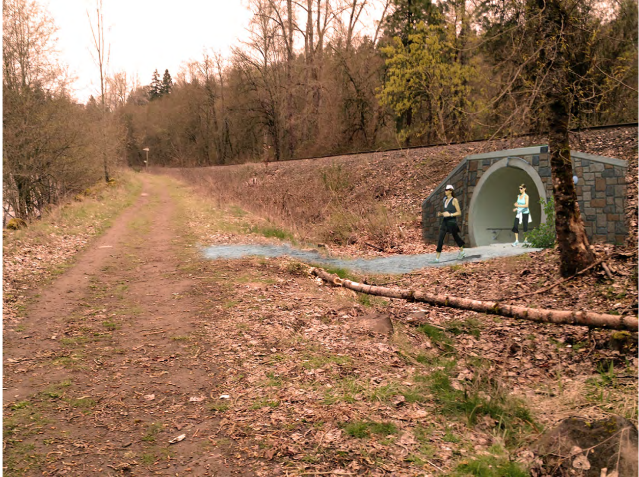
Figure 7: Artist's rendering of a culvert-type railroad underpass, downstream of the current terminus of the "Kodak Point" trail.
