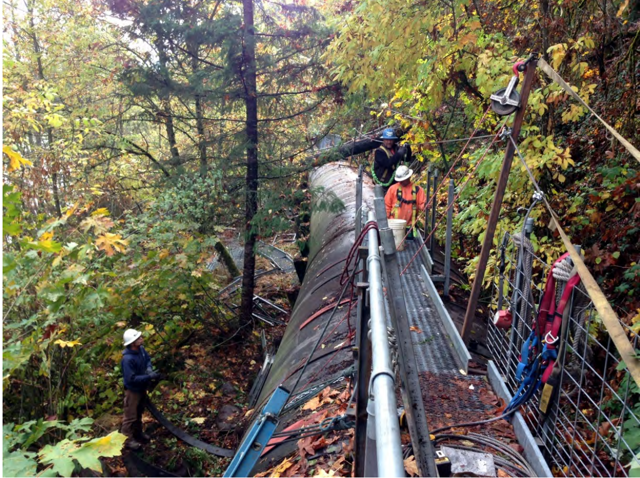
Figure 18: Crestline Construction crew working on catwalk repairs, November 2015.
